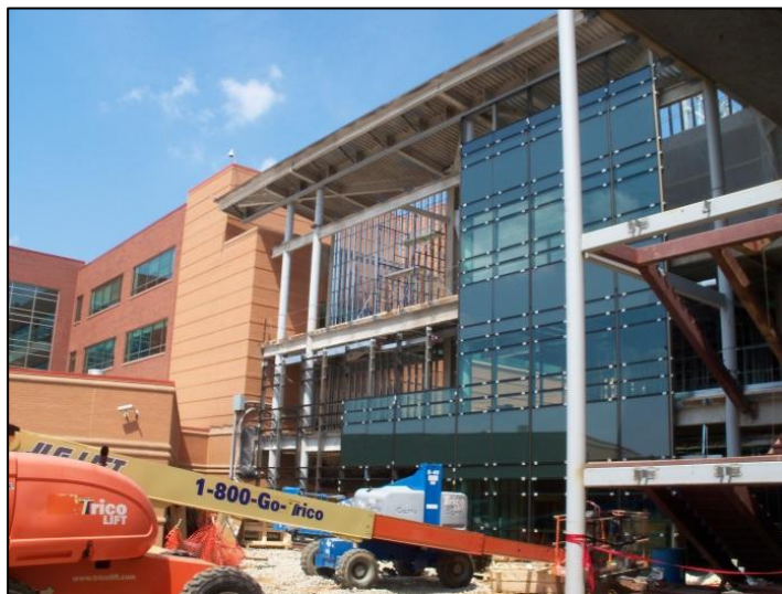
Figure 10 - View of west elevation curtain wall system under construction. The boom lift used during construction of the façade system can be seen at the bottom of the photo. Personal photograph taken by Chris Pozza.
