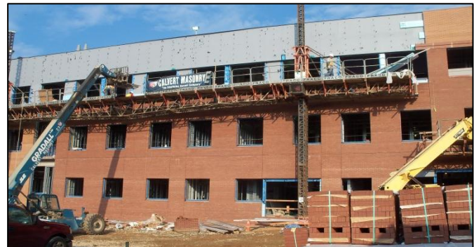
Figure 9 - View looking at east elevation. Fraco Lifts are used around exterior to provide efficient flow of construction along a large percentage of elevation at a time. Materials are lifted into place with a boom lift. Personal photograph taken by Chris Pozza.
