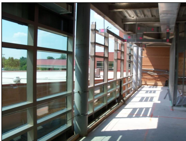
Figure 11, left – Interior view of west elevation curtain wall system under construction. Personal photograph taken by Chris Pozza.
