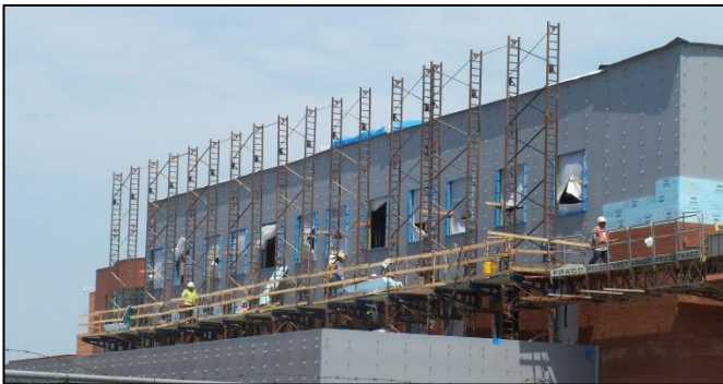
Figure 8 - View looking at southwest elevation. A MasonKing lift is required in areas where work is done above rooftops. These lifts have to be simultaneously cranked by hand to be lowered or raised. Personal photograph taken by Chris Pozza.
