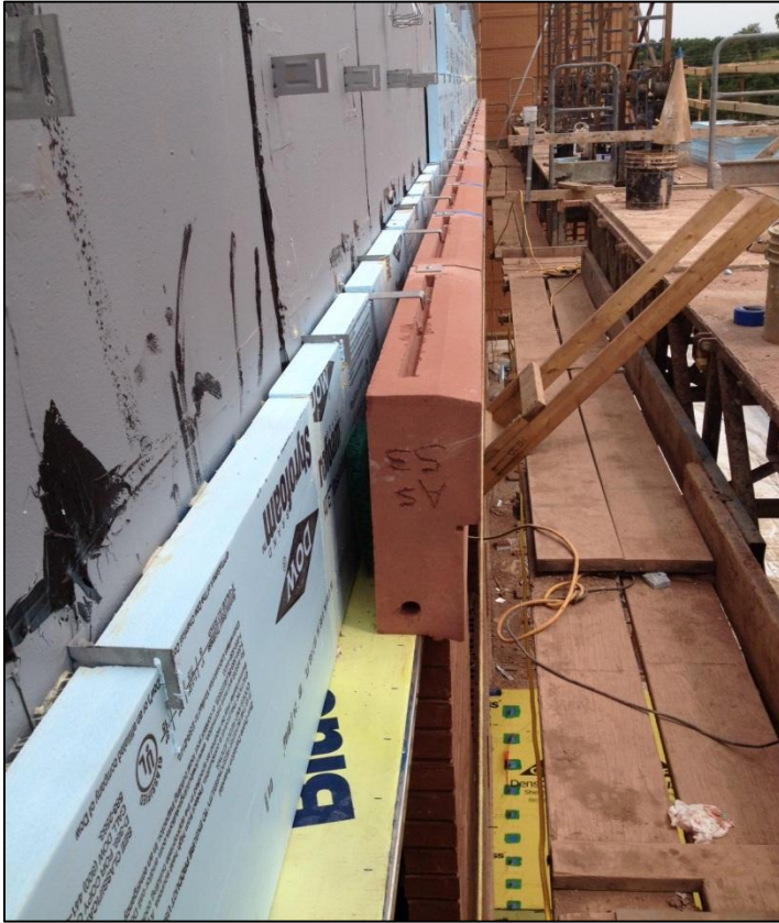
Figure 4 - Precast concrete can be seen above which make up the accent band along with east elevation. Personal photograph taken by Chris Pozza.
